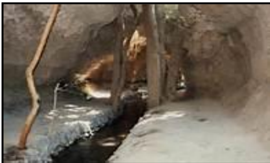
Underground irrigation system
